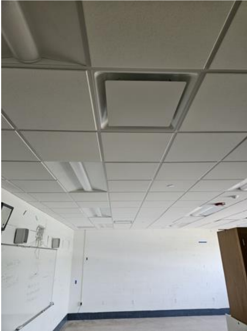
Diffusers Installed
