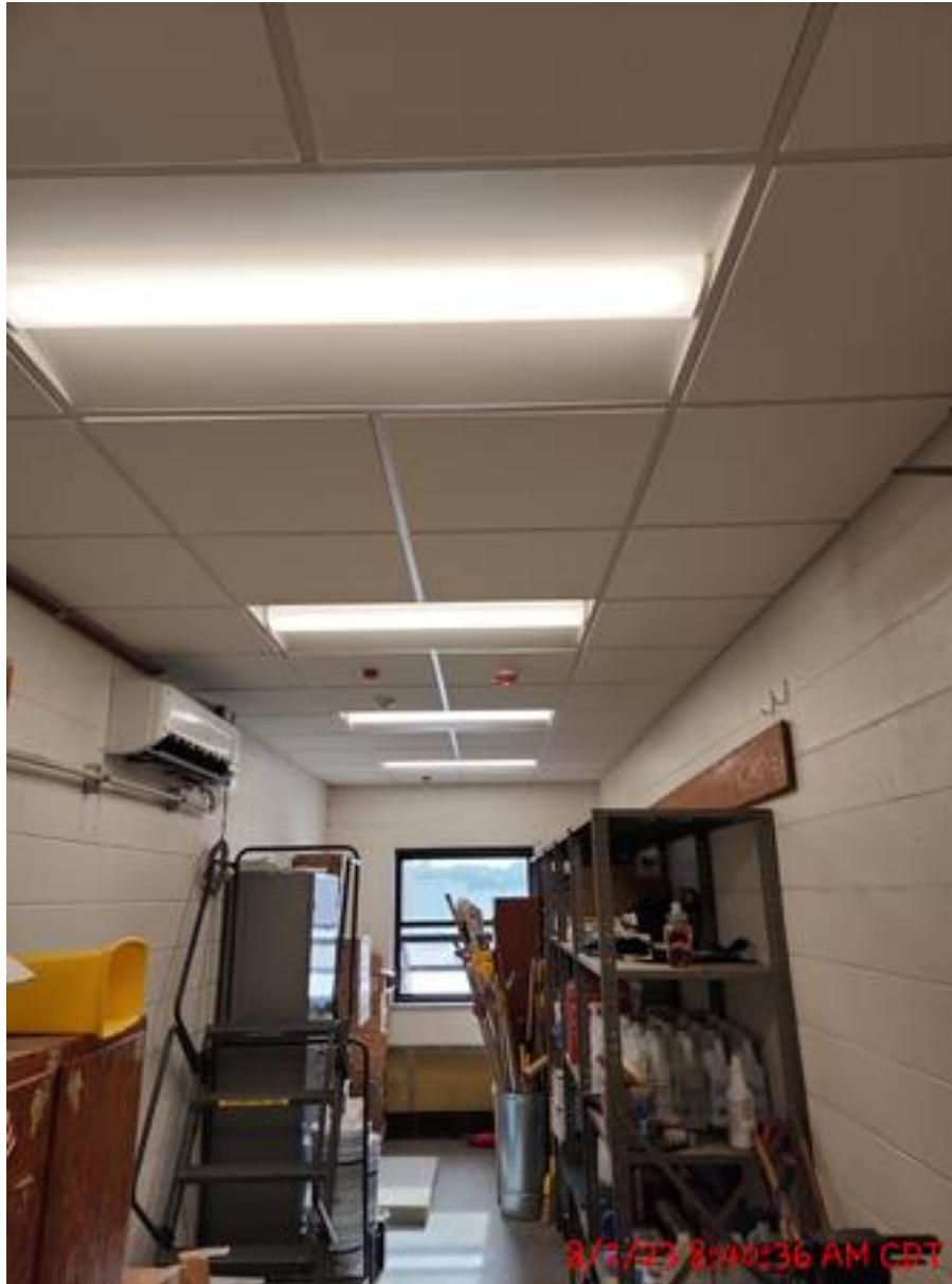
Complete: Lights and Fire Alarm Devices
