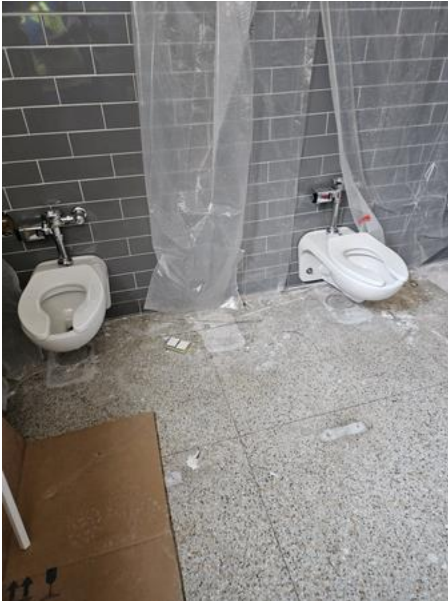
Water Closets Installed
